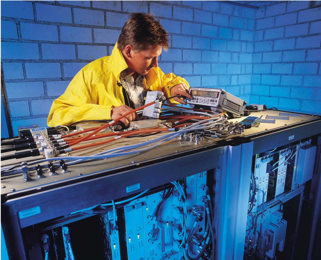
Installing a mobile radio base station with NRT (photo 42667)
